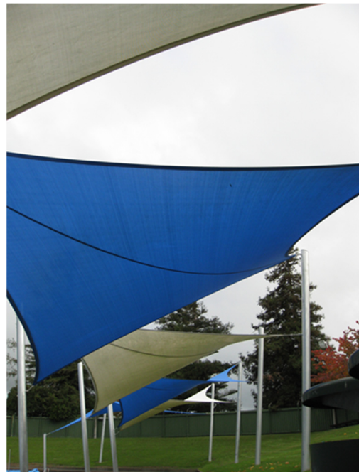
Figure 33: This view illustrates the openness of the shade to the sky (and to diffuse UVR)
