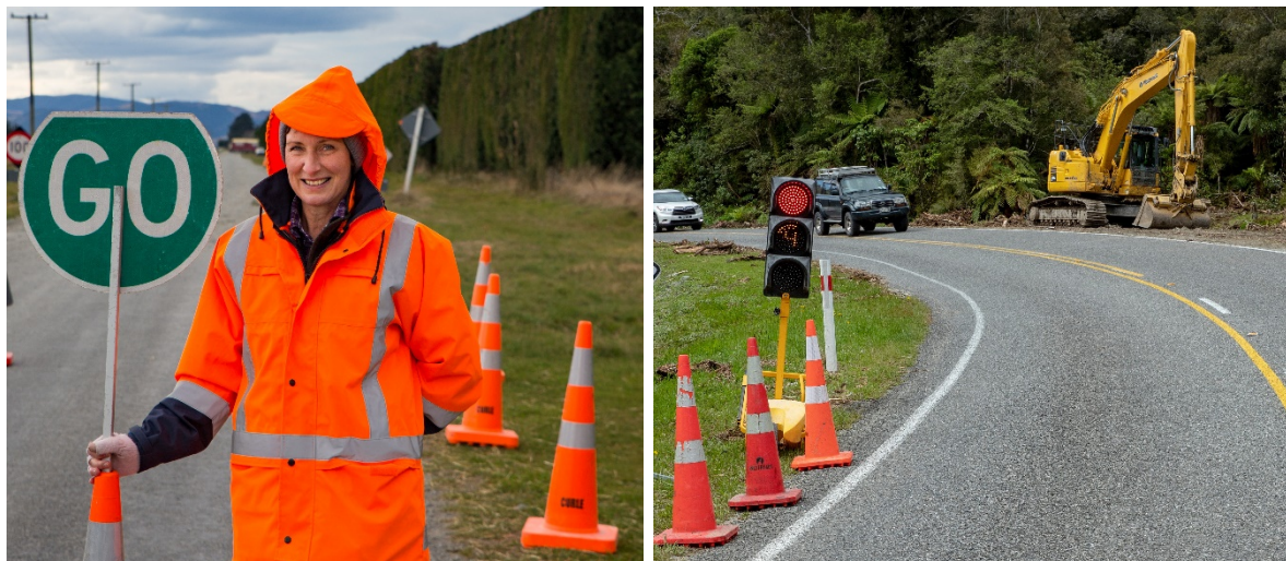
person wearing PPE (left) and substituting in traffic lights to minimise risk (right)
