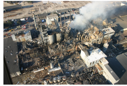
Vorderbrueggen, J. B. (2011). Imperial sugar refinery combustible dust explosion investigation. Process Safety Progress , 30(1), 66-81.
