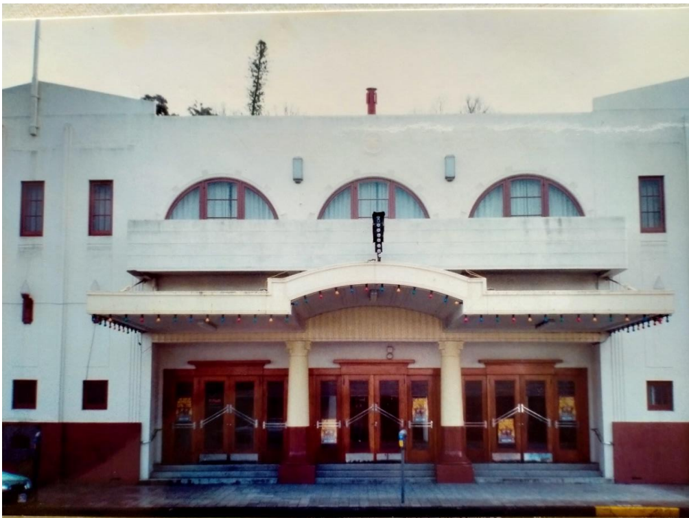
Figure 8. Municipal Theatre, built 1937 (119 Tennyson St, Napier. John Watson, architect. Photograph by Paul Moon).
