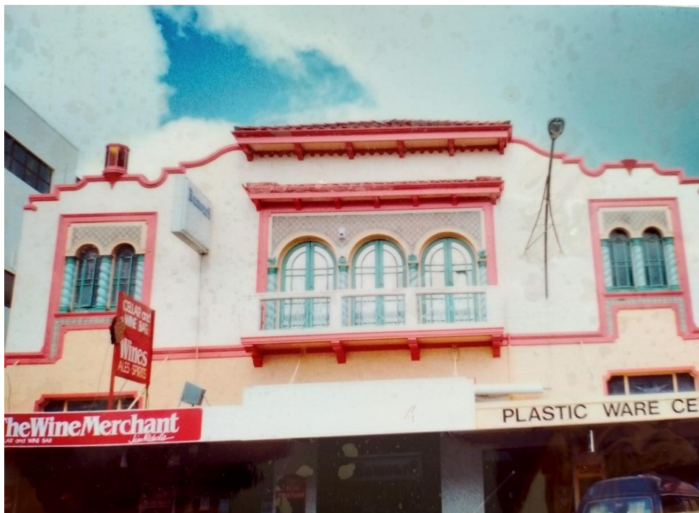
Figure 10. Gaity Theatre, built 1931 (88 Dickens St, Napier. Walter Finch and Alexander Westerholm, architects. Photograph by Paul Moon).
