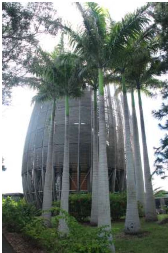
Renzo Piano-designed Tjibaou Cultural Centre, Noumea, photo by Elizabeth Thomson
