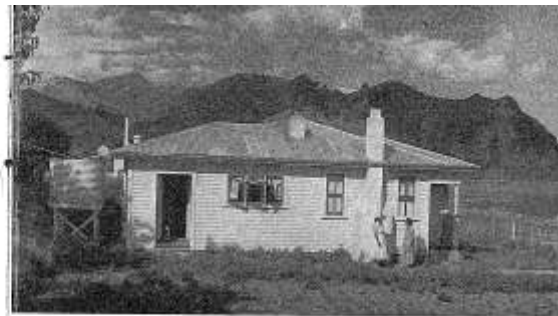
The house and bath at Tokomaru Bay by the Department of Maori Affairs for Mr. Kaiti and Mrs. Hargreaves Collier. (source: jones 2009).
