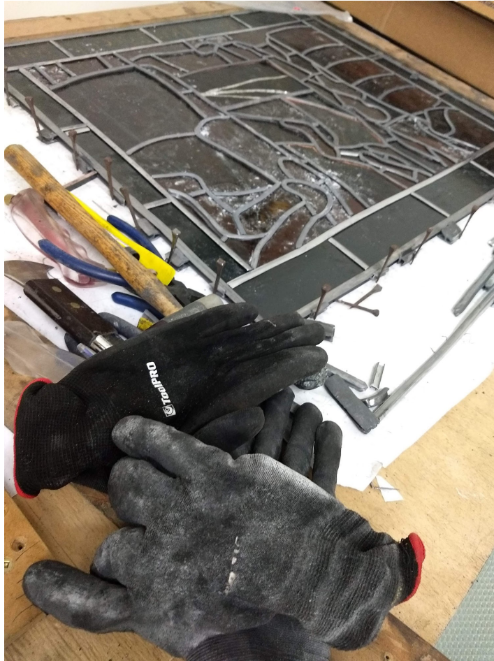
Figure 11. The window laid out completely with lead. The tools visible are those used for leading, and the gloves to prevent too much exposure to the lead
