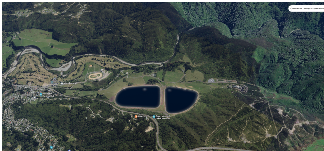
Figure 5. Aerial view of the Te Marua reservoirs (Stuart Macaskill Lakes) (Source: Bing Maps (Microsoft), 2025).
