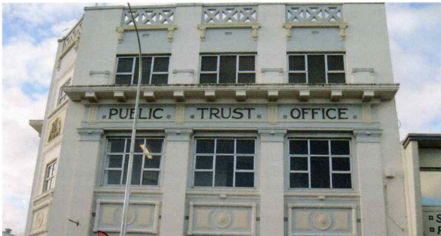
Figure 5. Public Trust Building from Perry Street. Mark Pacey
