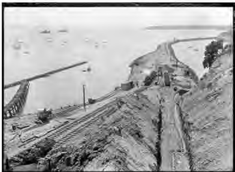
Reclamation work at Campbells Point, 1927. Auckland Libraries Heritage Collections I-W0778.
