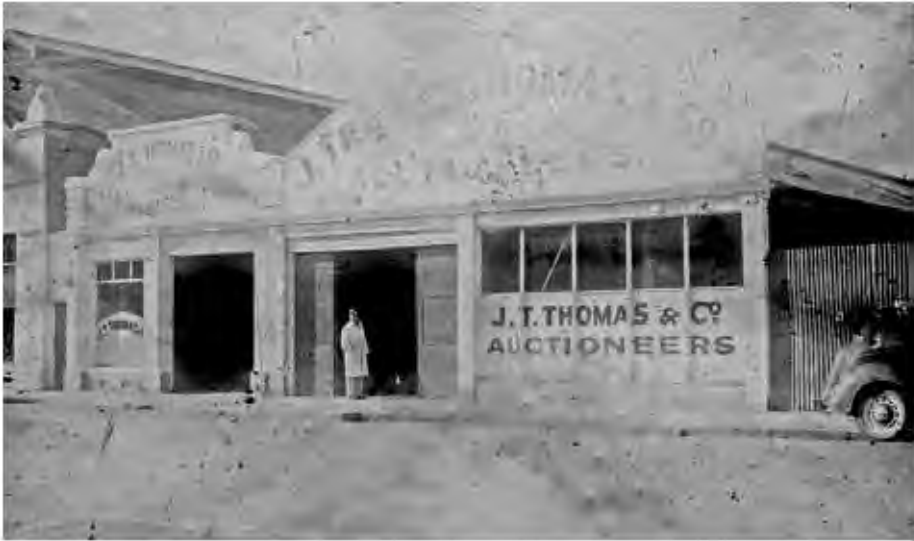
Figure 4. John Trevor Thomas' business premises on Tancred Street, Ashburton c. 1950s.
