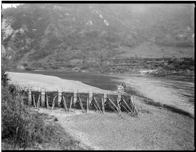
Eel or fish weir at Pungarehu, on the banks of the Whanganui River. Whole-plate collodion silver glass negative. Photographer: William Harding, between 1856 and 1889. Ref. 1/1-000483-G. Alexander Turnbull Library, William James Harding Collection.
