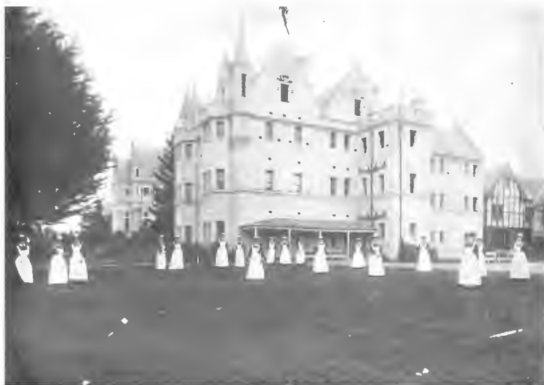
The imposing buildings at Seacliff [archives reference: DAHI 20271 D266/520a].
