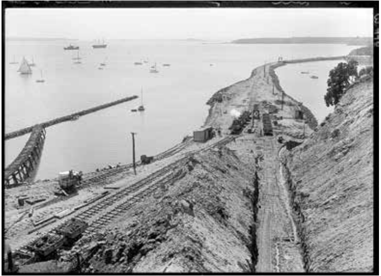
Reclamation work at Campbells Point, 1927. Auckland Libraries Heritage Collections 1-W0778.
